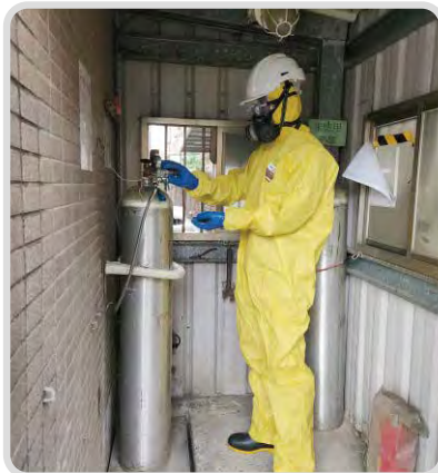
Gas supply shut off
