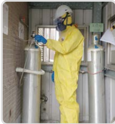
Gas supply shut off
